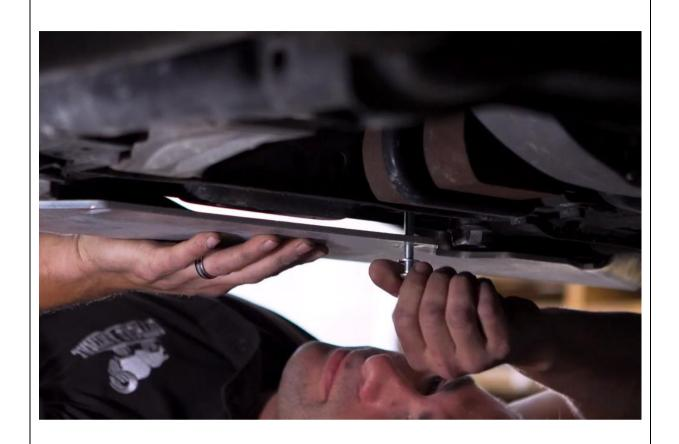
6. Fit M8 Button head cap screws to rear of bash plate in factory threaded clips.
